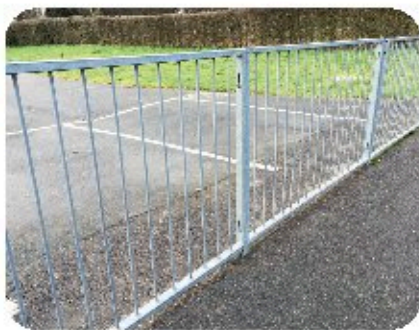
Flat top fencing
